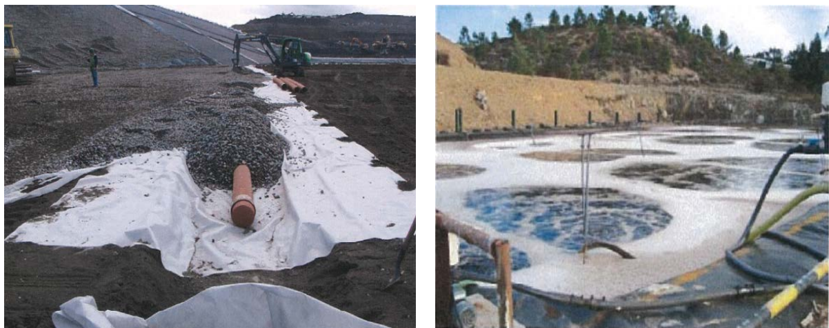
Figure 4.2-96 Example of installation of Leachate Collect Pipeline (Left) and Leachate Treatment Ponds (Right)
